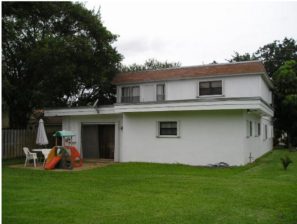
4. VIEW NORTHWESTERLY OF NORTHERLY ADJACENT RESIDENCE LOCATED AT 733 SW 4 STREET
